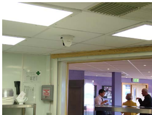
'KitchCam' – one of the kitchen ceiling mounted Elmo PTC450's (Photo is of view through server hatch to restaurant)
